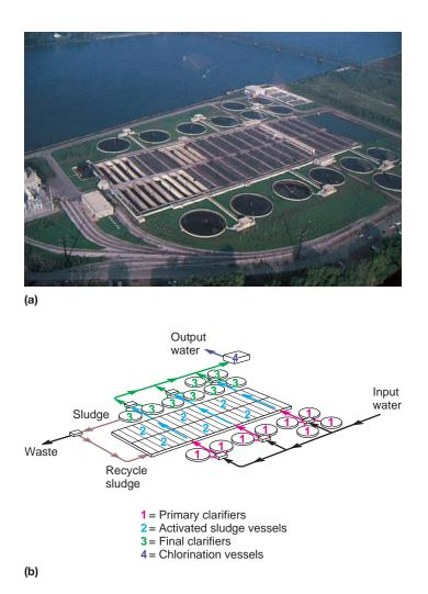
**Figure 41.4** An Aerial View of a Modern Conventional Sewage Treatment Plant. Sewage treatment plants allow natural processes of self-purification that occur in rivers and lakes to be carried out under more intense, managed conditions in large concrete vessels. (a) A plant in New Jersey. (b) A diagram of flows in the plant.
